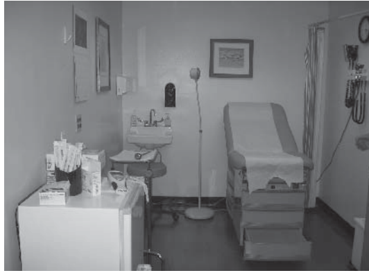
Partial view of one of the Exam rooms in the recently renovated clinic space.
